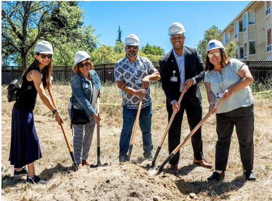
Providence Northern California's Community Health Investment team breaks ground for supportive housing in Napa with leaders from Providence Queen of the Valley Medical Center.
