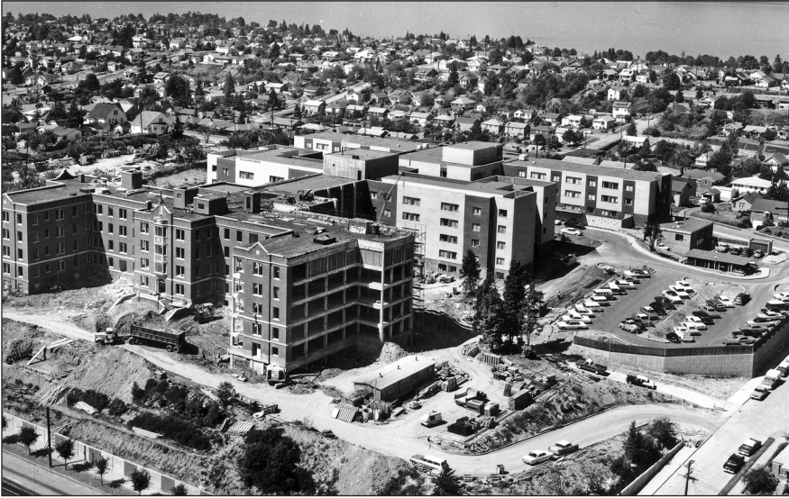
View west shows completed SJR in background; west portion of the Mount completed in center; and east portion of Mount under construction, 1967. Image #140.A3.7
