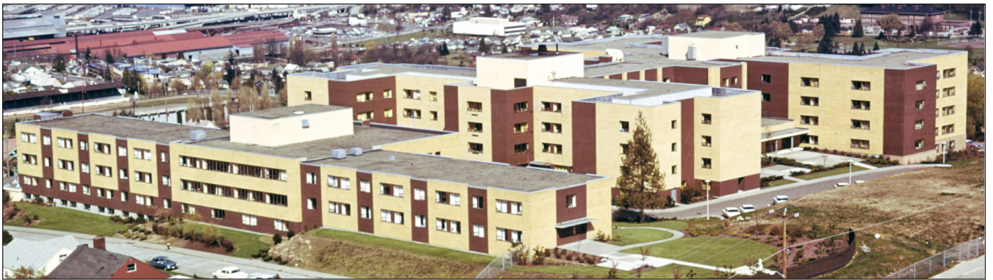
View northeast after project completion shows both SJR (foreground) and the Mount with unified architectural style. Image #140.A4.31
