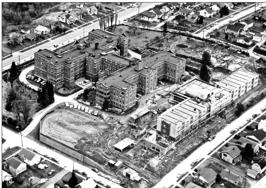
View southeast shows SJR under construction at right, 1965. Image #140.A3.2
