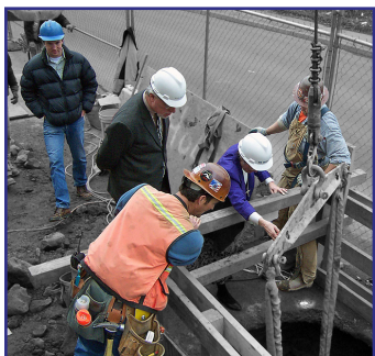
Sr. Rosalie dropping a medal into a concrete pour
